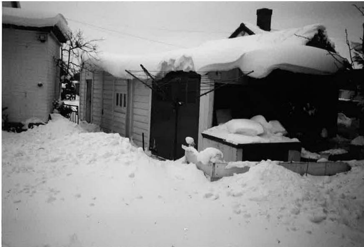
2 View of demolished garage from rear
